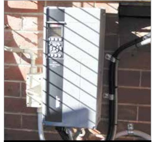
VSD unit maintains temperatures when operating at part load
