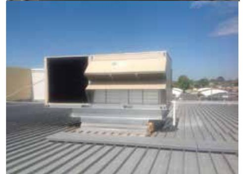
Roof curbs eliminated the need for additional penetrations and external ducting
