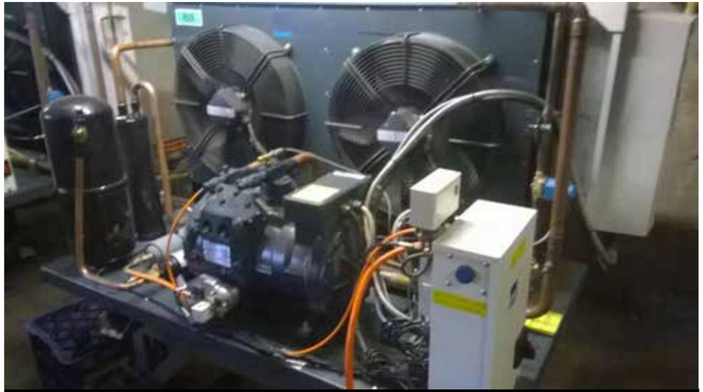
The soft start feature of the Variable Speed Drive reduces compressor starting current by up to 40%.
