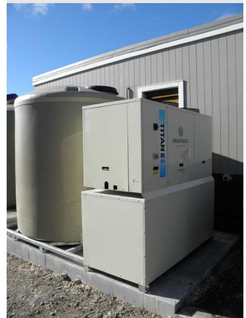
Snapchill runs off peak storing the cooling energy until needed as well as providing free 82°C hot water
