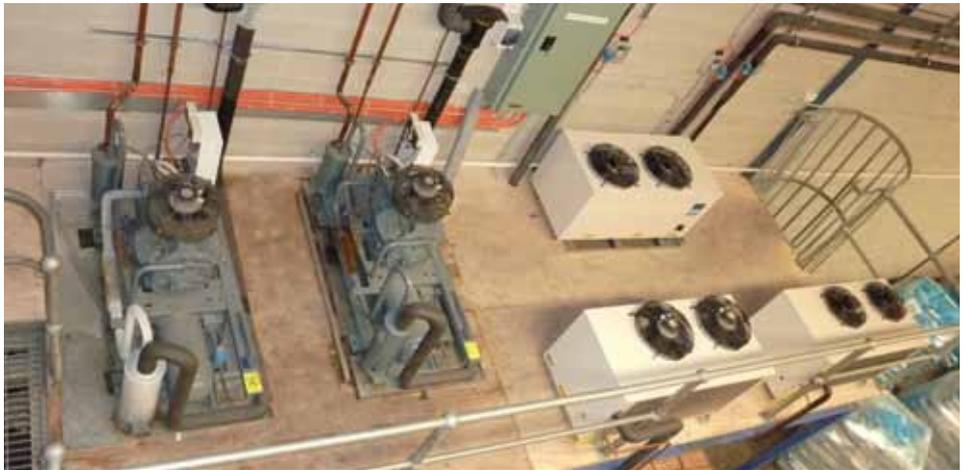
A view of the mezzanine level which houses the two 15 HP Dorin basic units and three Kirby Polar Pack units.
