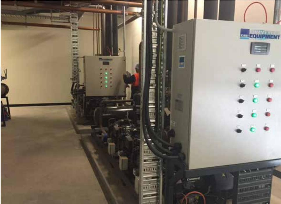
Due to the size of the refrigerated space the initial pull down to temperature did take some time but was expected due to the heat in the walls and concrete. With the heat removed, the room now maintains stable temperatures, with many of the compressors on each rack often cycled off onto standby.
