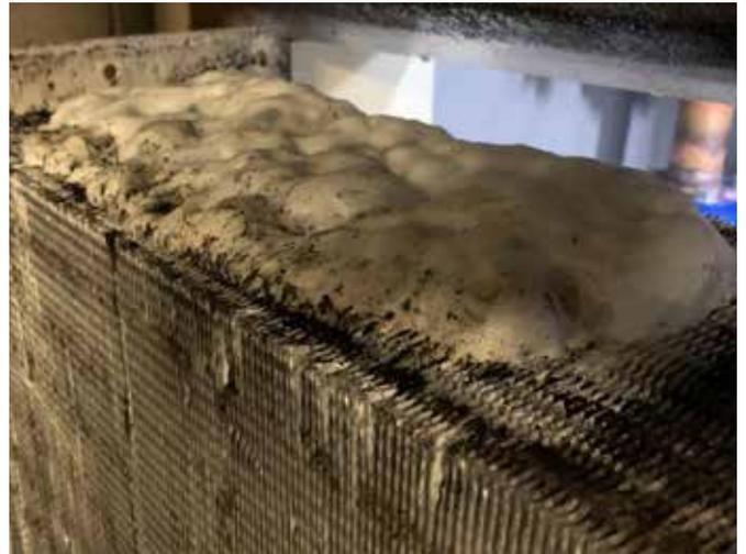
Image 4: Spraying onto the coil initiated the foaming action, pushing out and removing the hard carbon.
