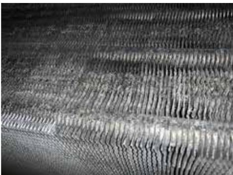
Image 1: Hard carbon contamination was quite evident not only on the surface of the coil, but also deep within the fins and rows.
