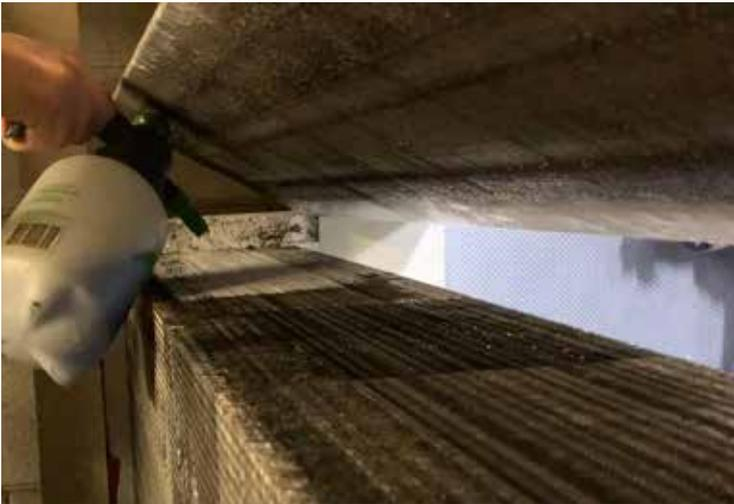
Image 3: Initially Viper Brite was applied on a small section from the left side on the air onto the coil.
