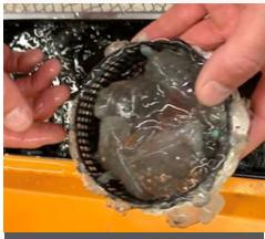
If the refrigerated case and condensate pump was not proactively cleaned, this biofilm evolved into thick sludge
