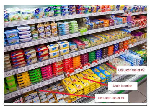
The customer was shown the correct way to install the product for these cases i.e Install 1 x Gel Clear tablet on the high end of either side of drain entry point. This allowed the tablet to slowly dissolve and coat the condensation path.
